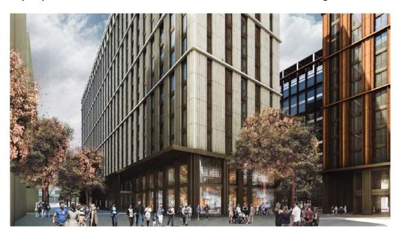
The ground floor facades to both developments would have glazed frontages set within a regular rhythm of double height columns which would allow visual permeability into the ground floor commercial units whilst creating an interesting articulation to the facade. The lower levels have been designed with all back of house activities located deep within the floorplate to ensure maximum levels of
